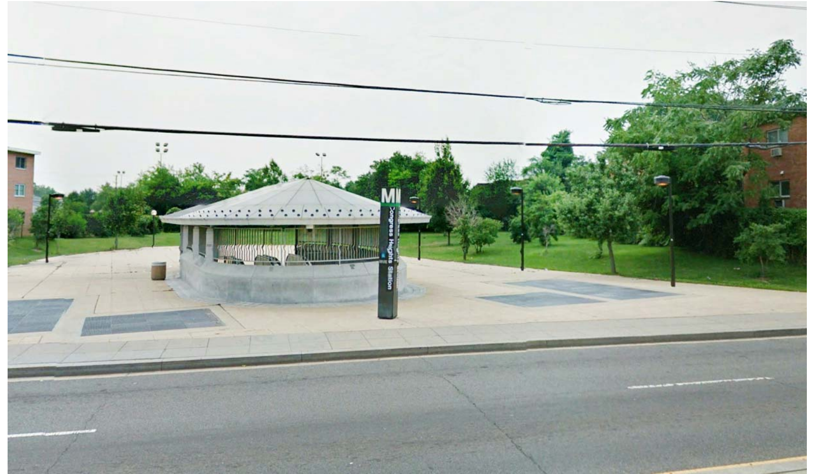
View of metro entrance from across Alabama Ave.
